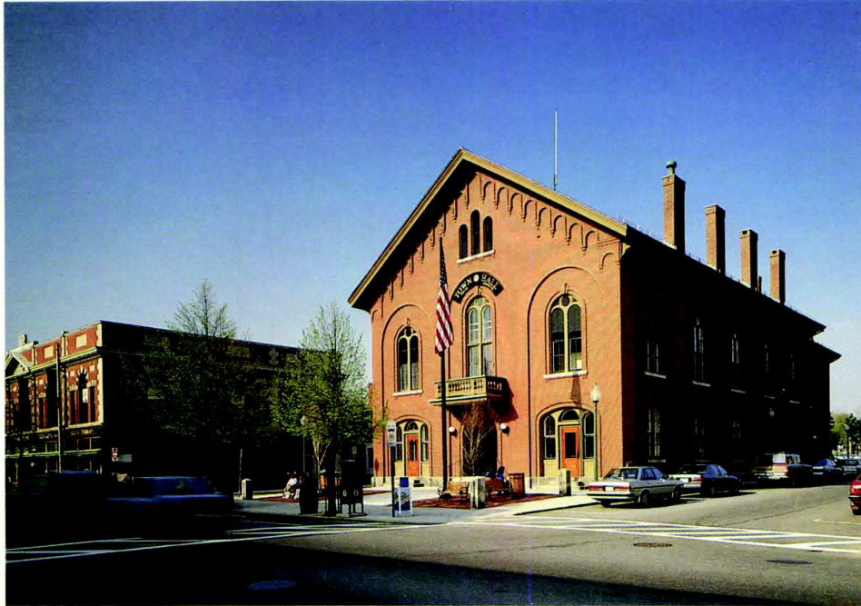
Town Hall occupies a prominent site on Main Street in downtown Andover.
