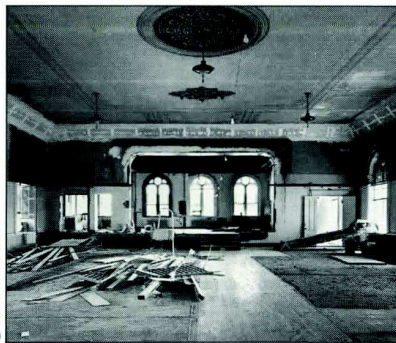
The auditorium before $2.1-million restoration.
