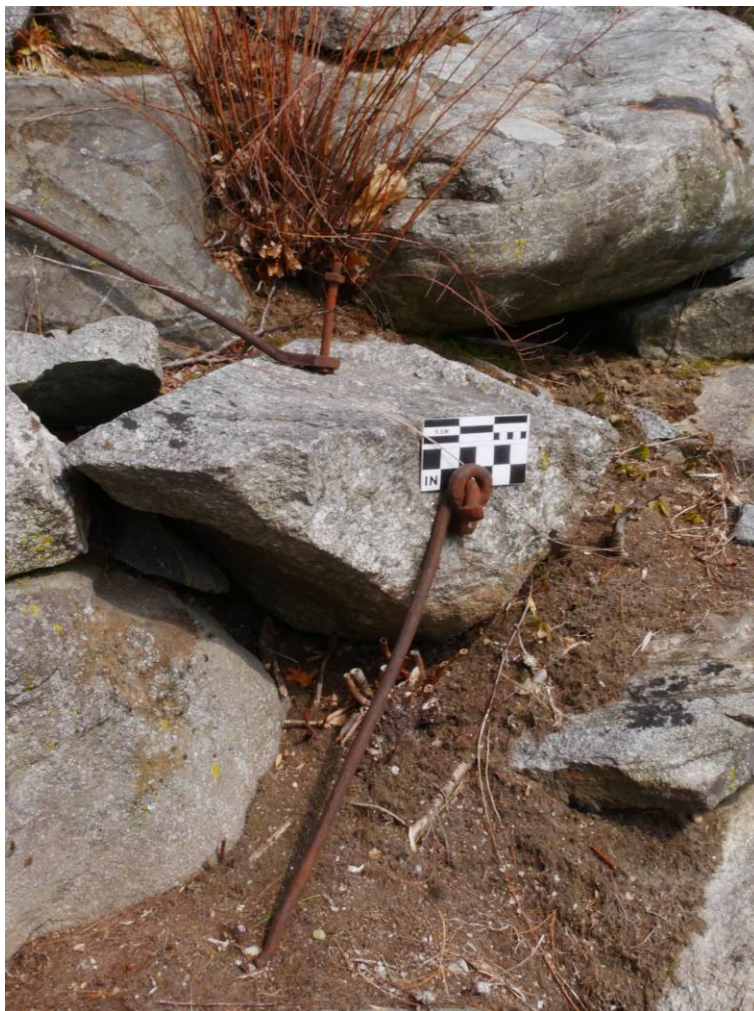
Figure 6 – Metal rods attached to the eyebolts use to secure the “summer house” a small building on the mound in the 1930s.
