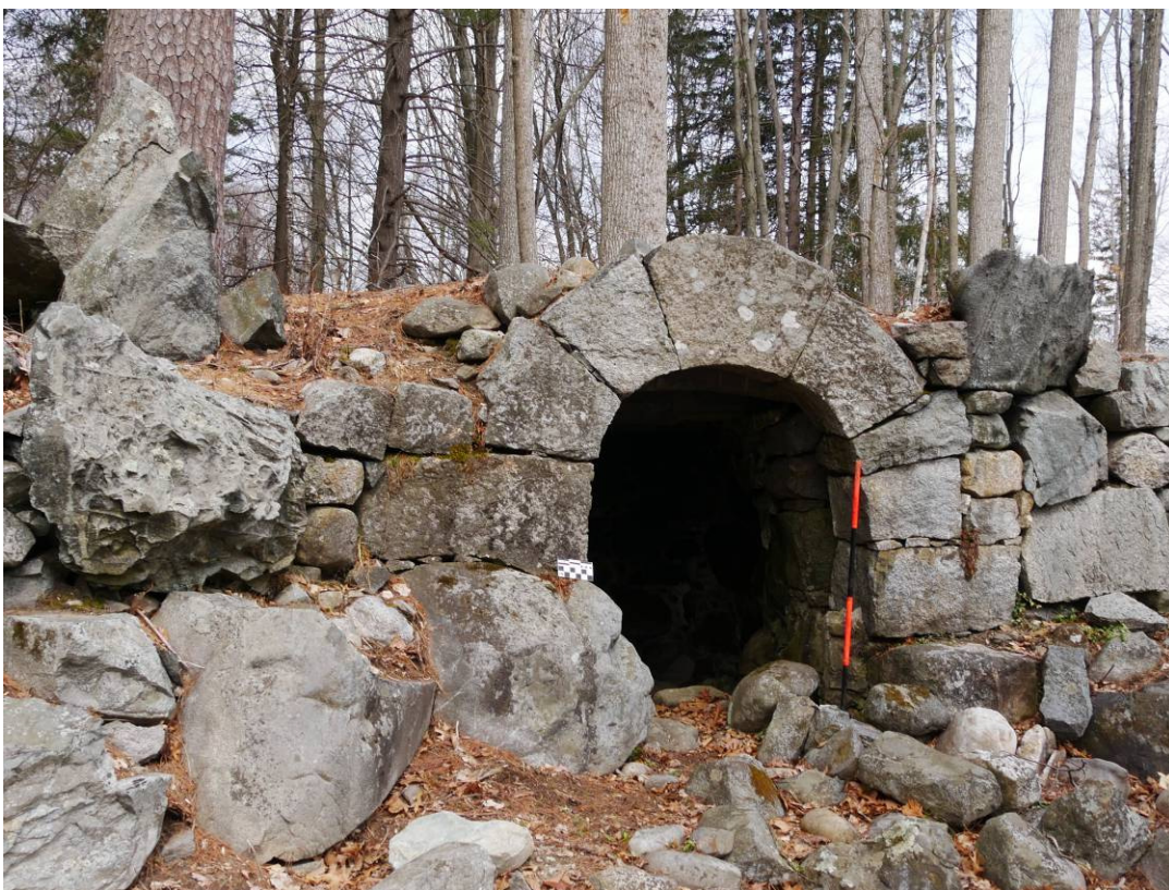
Figure 9 – Plug and feather method quarried granite arch entrance of the south grotto. Another one of the sculpted (differentially weathered) stones is seen to the left of the entrance.
